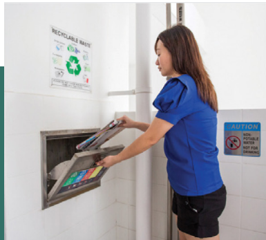
SEPARATE CHUTES FOR RECYCLABLE WASTE
