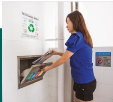
SEPARATE CHUTES FOR RECYCLABLE WASTE
