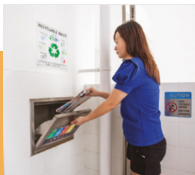
SEPARATE CHUTES FOR RECYCLABLE WASTE
