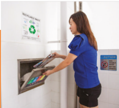
SEPARATE CHUTES FOR RECYCLABLE WASTE
