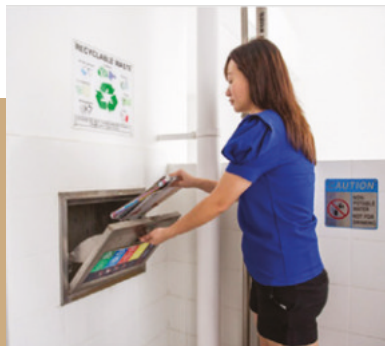
SEPARATE CHUTES FOR RECYCLABLE WASTE
