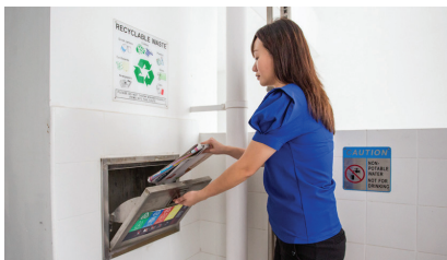
Separate chutes for recyclable waste
